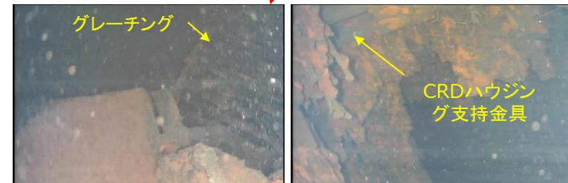
Situation of PCV bottom (Unit 3)
